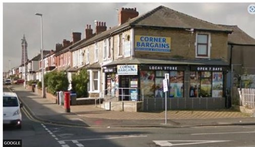
Corner Bargains on Caunce Street, Blackpool, as handed a council closure order
